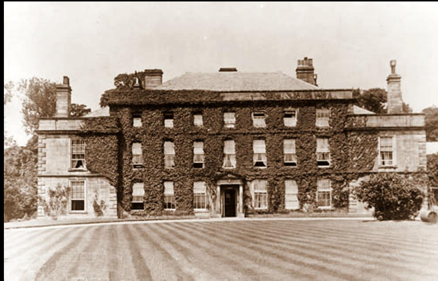
Manydown House, before demolition in 1965.
